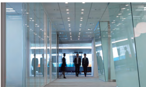
Glass wall with slope angle of six degrees, which is totally different from conventional vertical glass walls
